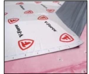
**Step Five:** For general sealing around penetrations, Firestone AP Sealant may be used. When full water tightness is required, terminate the V-Force Vapor Barrier Membrane with UltraFlash™ One-Part Liquid Flashing. Install a base coat, fleece layer, embedment coat and top coat per UltraFlash application guidelines.
