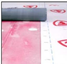
Position the membrane so that side laps are at least 3" (76 mm) and end laps are at least 6" (153 mm). Rolls must be staggered a minimum of 12" (305 mm). Begin application at the bottom of the slope and overlap in shingle fashion so the laps shed water.
