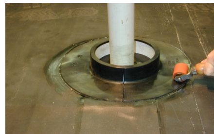
Roll QuickSeam Penetration Pocket flange with hand roller
