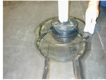
Apply Lap Edge Treatment at all lap edges
