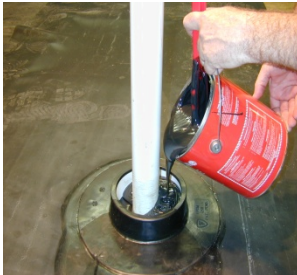
Fill QuickSeam Penetration Pocket with Pourable Sealer S-10 or FillGard M Pourable Sealer
