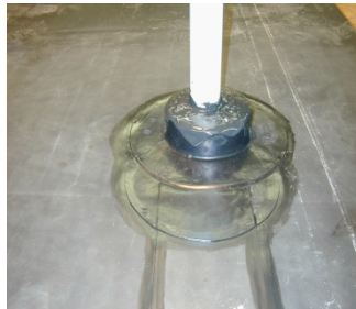
Completed QuickSeam Penetration Pocket
