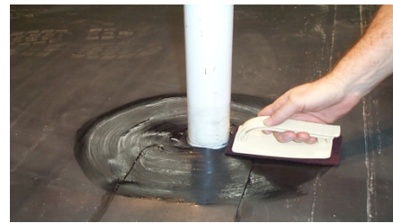
Scrub-apply primer to membrane & penetration
