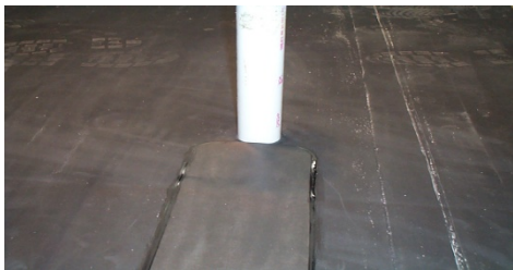
Repair membrane surrounding penetration as required.
